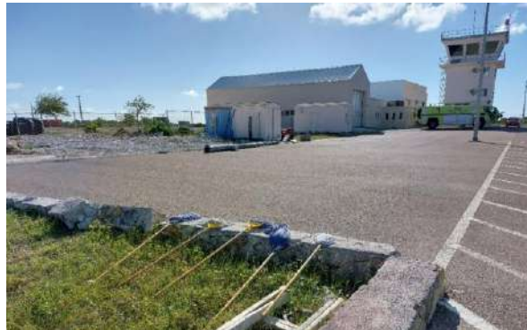
Cleaning practices are performed in a non-standard manner, which present hygiene risks
