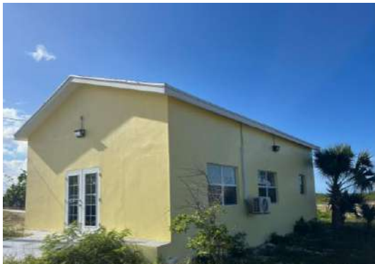
The main entrance of the 100m 2 terminal building, which was recently refurbished
