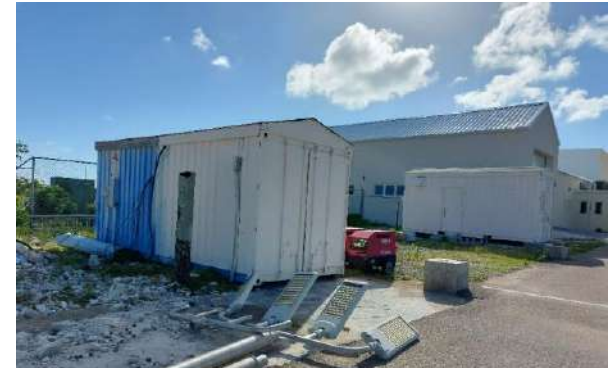
Construction materials are laid out throughout several areas, presenting threats to airport workers
