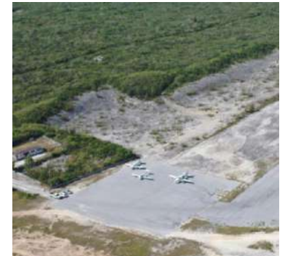
The airport currently does not have perimeter fencing
