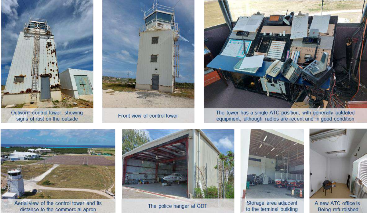
Figure 19. Current estate of tower and hangars
