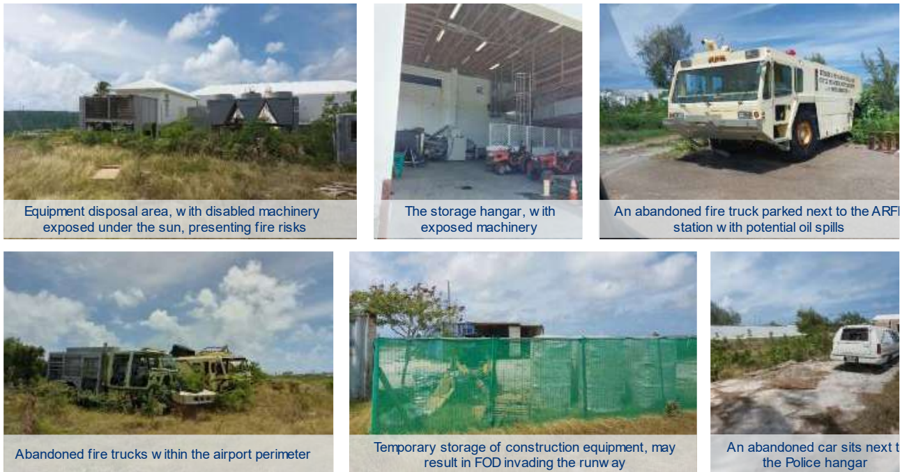
Figure 20. Current situation of machinery and equipment
