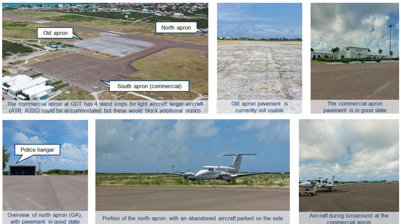
Figure 12. Apron images obtained during the site visit
