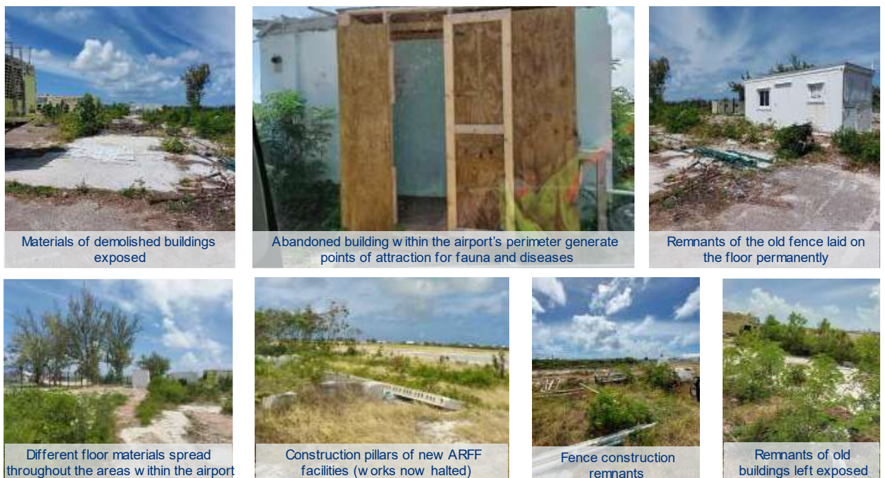
Figure 21. Current situation of old structures and buildings
