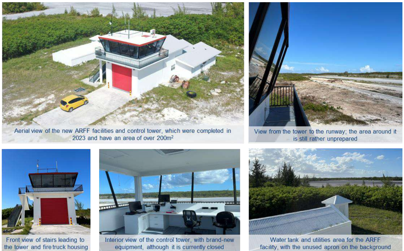
Figure 6. Current state of ARFF and control tower facilities and equipment
