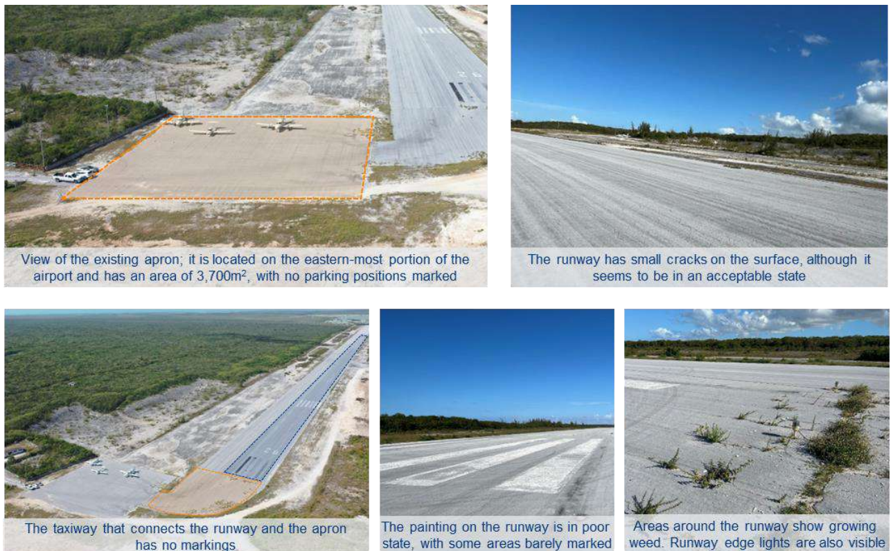
Figure 4. Runway, taxiway and apron images obtained during the site visit
