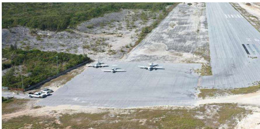
Figure 39. South apron aerial view
