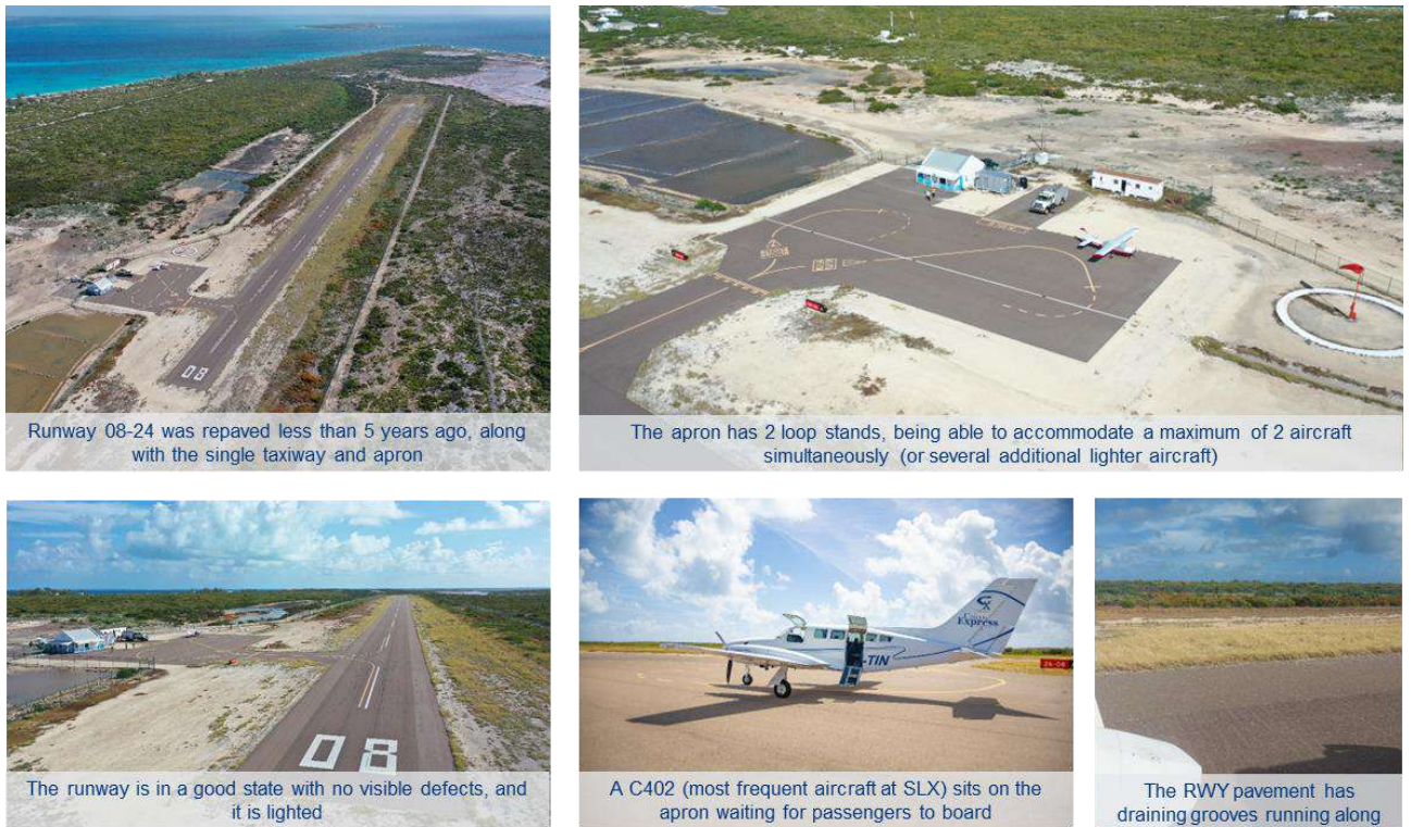
Figure 4. Runway, taxiway and apron images obtained during the site visit
