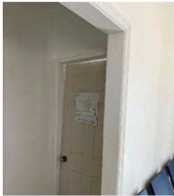
One of the terminal's bathrooms is unusable
