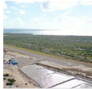
The adjacent saline ponds may flood the airport
