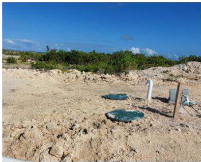
Unfinished construction areas with pipes and equipment exposed on the surface
