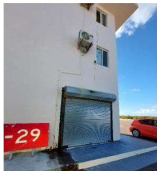
Spilled oil and other materials from brand new buildings
