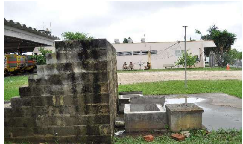
Example: Recycling water from ARFF trucks in Curitiba Airport (Brazil)
