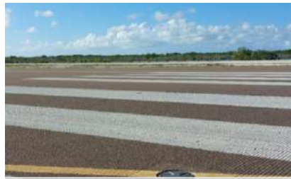
Horizontally grooves for water drainage
