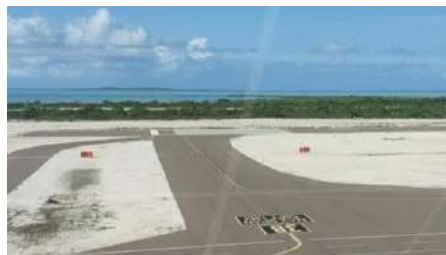
Taxiway A, connecting apron to RWY
