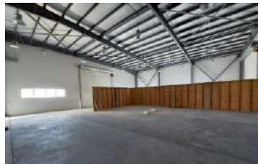
ARFF facility's interior w/o fittings
