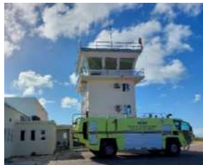
ARFF and control tower
