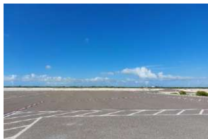
Apron pavement in good state
